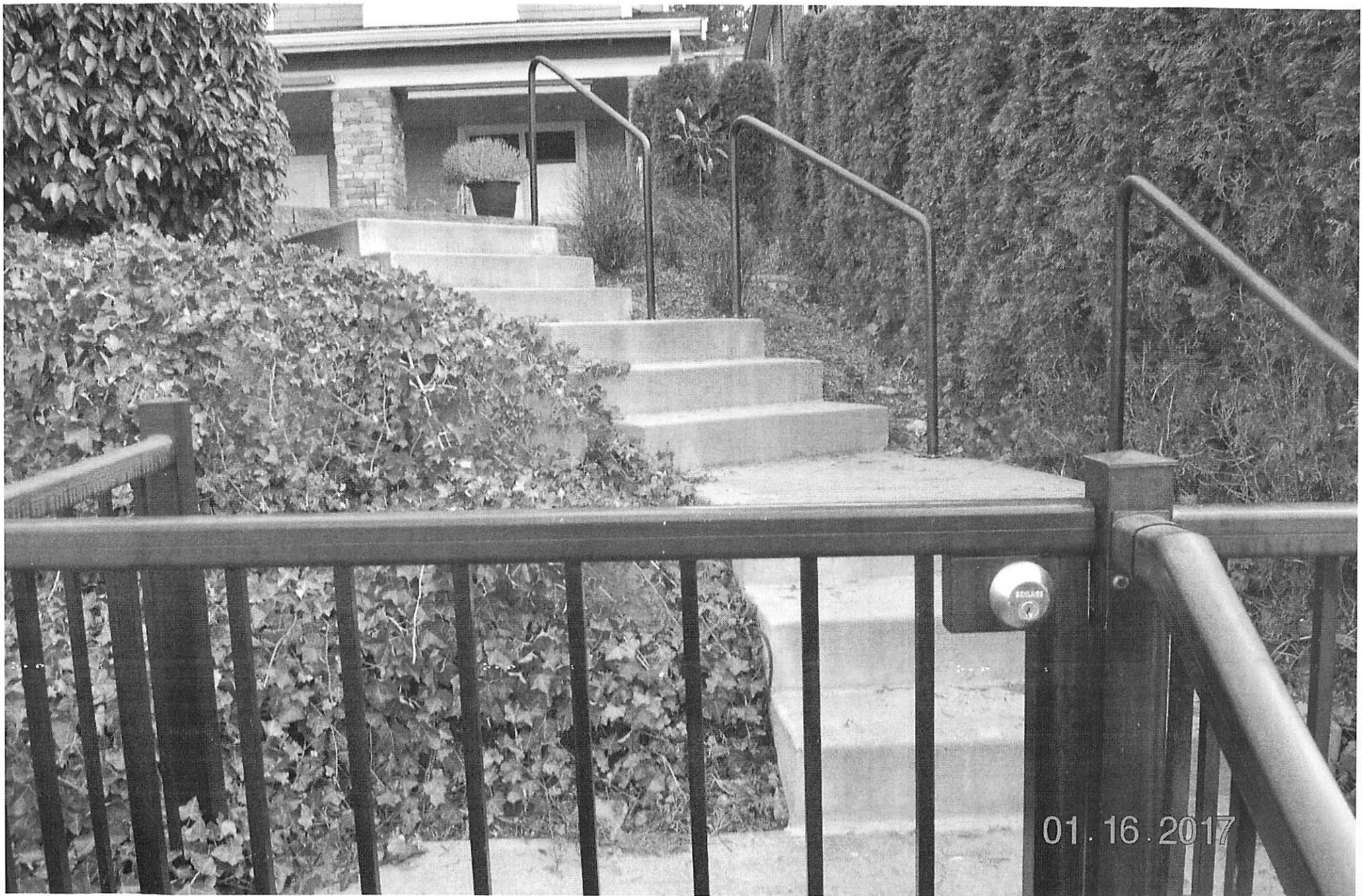
UP VIEW OF SB-597 Concrete Steps
