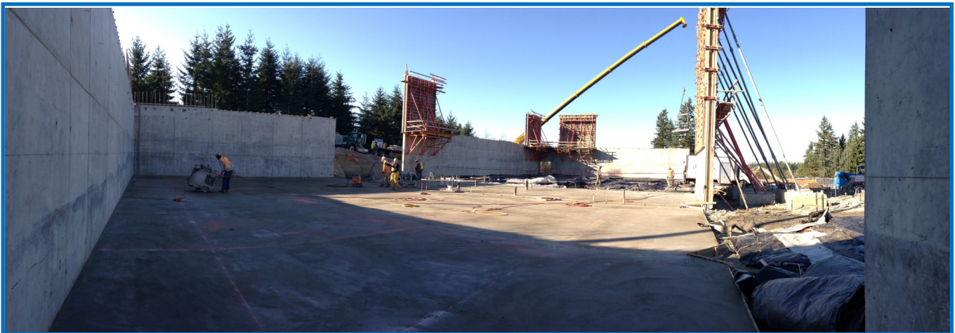
Above: Concrete pour for building slab in progress.
