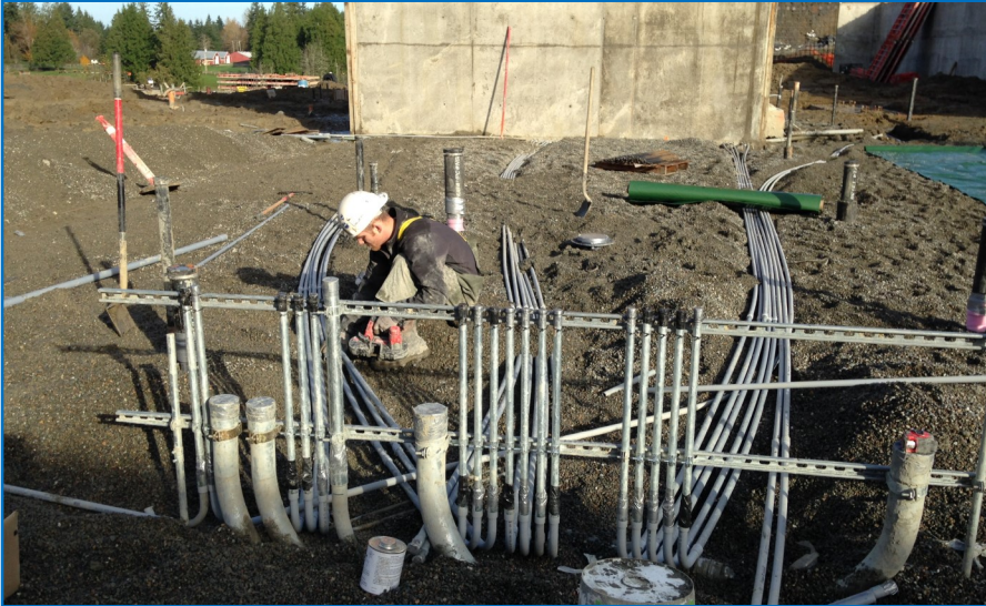
Utilities below the building slab
