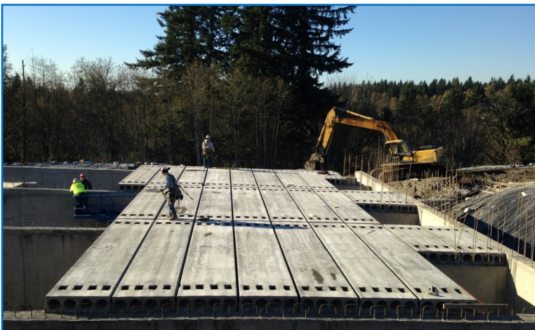
Placement of Hollow Core Planks
