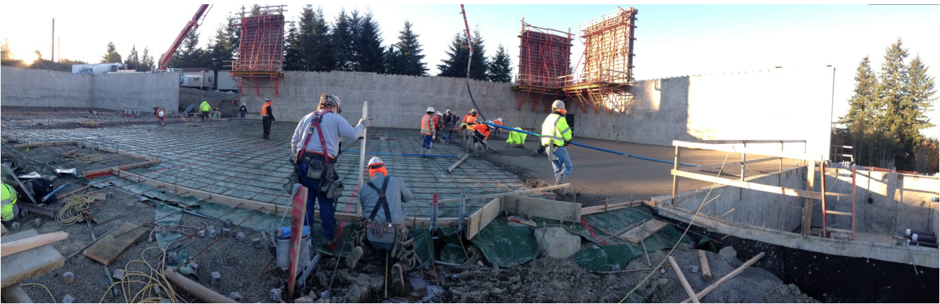
Above: Concrete pour for building slab in progress.
