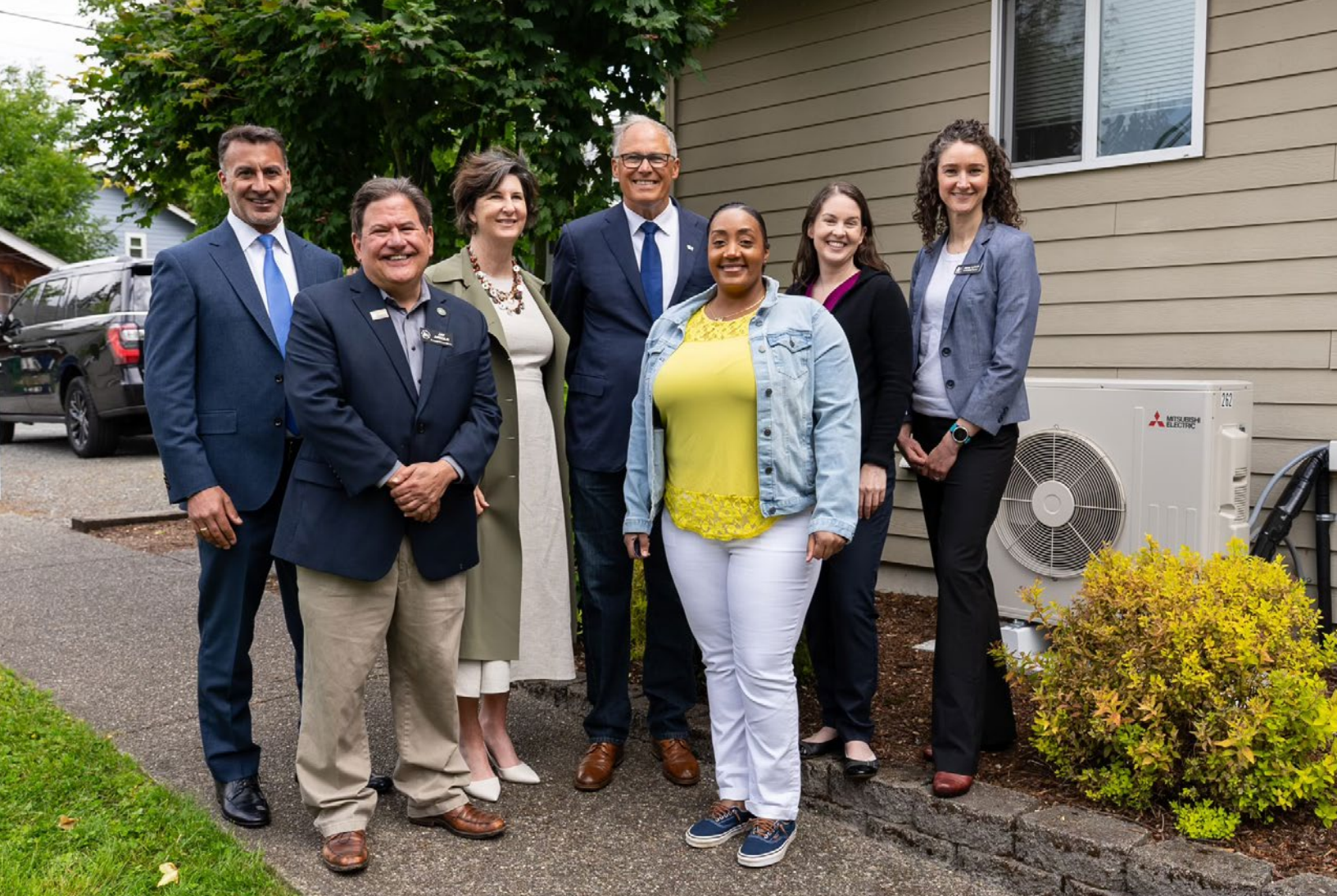
Tour of heat pump installations at Acres of Diamonds in Issaquah, 2024
