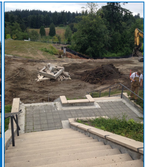
Below: Demolition of stairs from the upper plaza.
